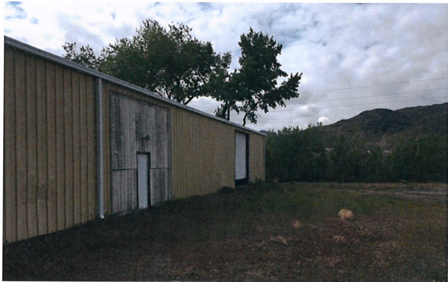
Existing industrial building
